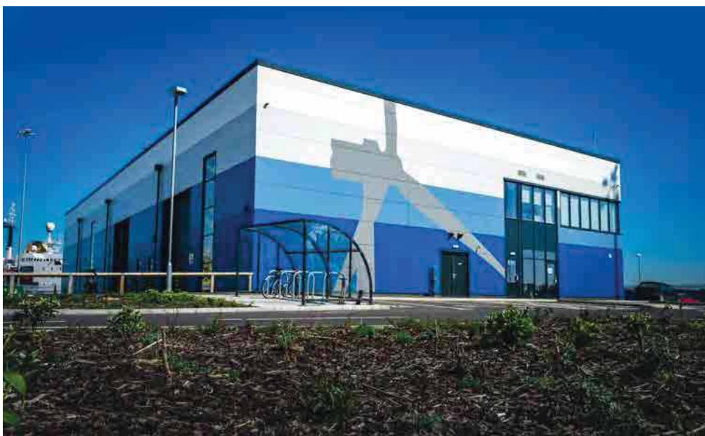
Galloper Operations and Maintenance base
