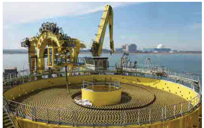
Export cable spool for Galloper Offshore Wind Farm during installation
