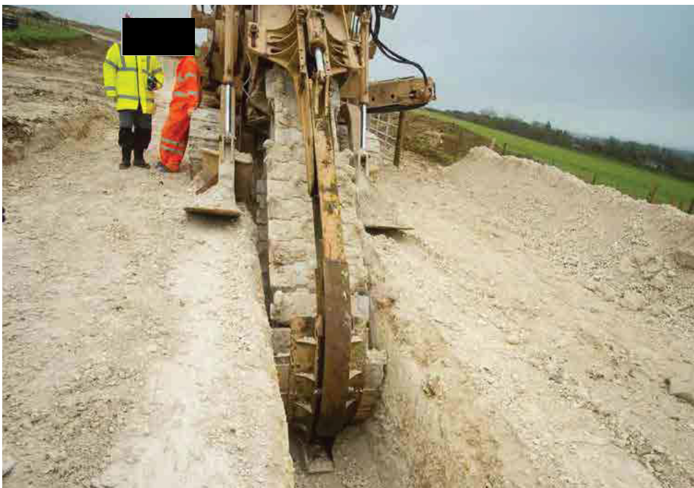
Open cut cable trench excavation
