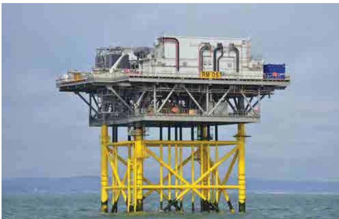
Offshore substation at Rampion Wind Farm
