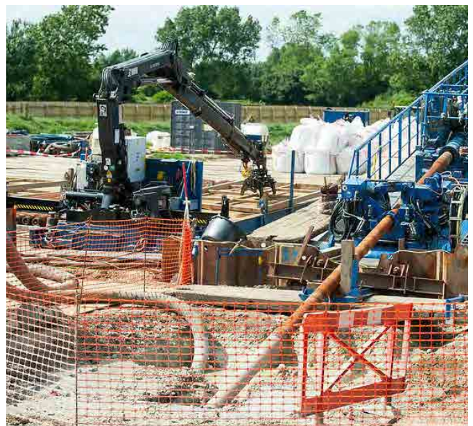
Horizontal directional drilling
