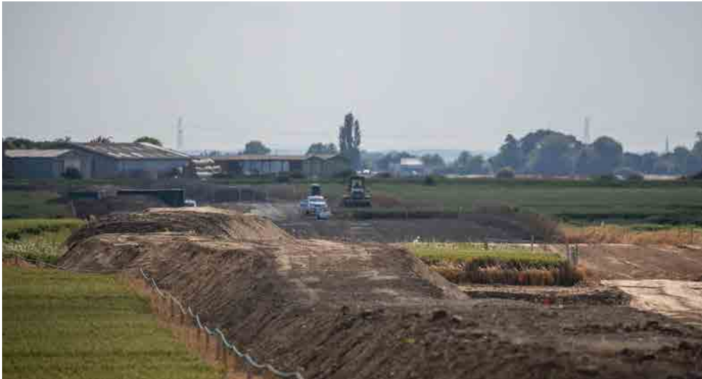
Example of soil storage during construction
